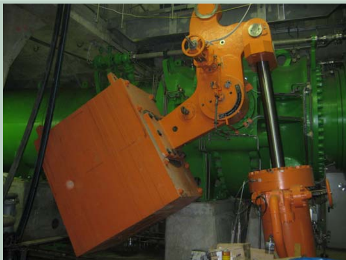
Predturbinski ventil 14. september 2009
